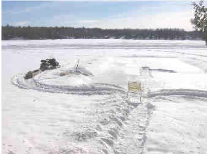
ice auger and our fire pump. It was a cold blustery day, the appropriate hole was drilled, the intake hose installed on the pump, the hose hooked up and the pump primed. Time to start the pump, it wouldn't fire, pulled the spark plug tried some more but no no avail, thus to plan B. Disconnected the pump, rolled up the hose and pulled the primer hose and brought them into the basement to thaw out. Back to the power auger with which I enlarged the
